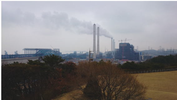
FIGURE 5: Infrastructure of the Dangjin power station.
